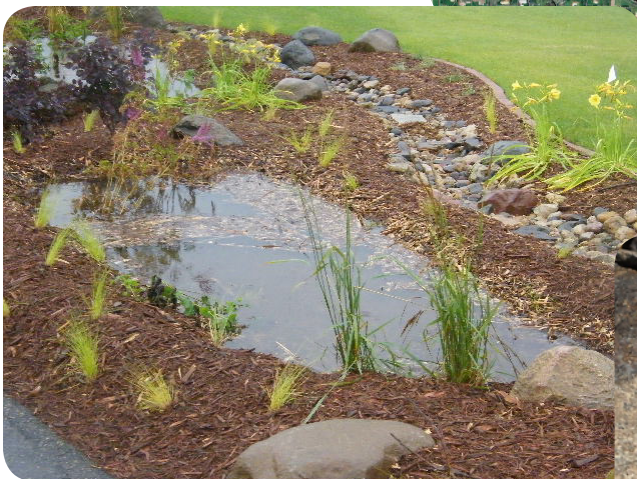
Above: Rain gardens in the new landscaping project capture runoff and soak it into the ground.
