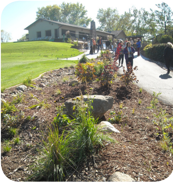
Above: A rock creek bed leads downhill from the club house to a series of rain gardens.
